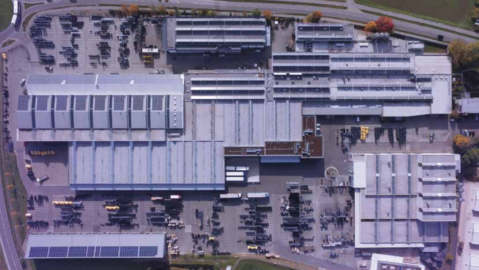
The KESSEL plant Lenting (Germany)
