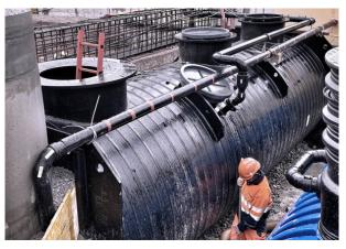
Installation example grease separator EasyClean ground Auto Mix & Pump NS 30
