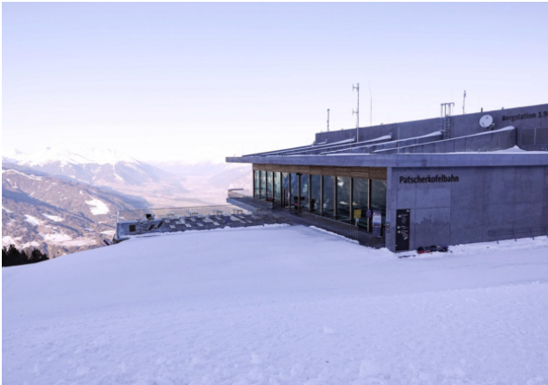
Restaurant 'Das Kofel' in the mountain station. (Source: KESSEL)
