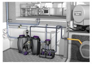
Installation example: Grease separator EasyClean free Auto Mix & Pump NS 15 with lifting station Aqualift F XL (Source: KESSEL)
